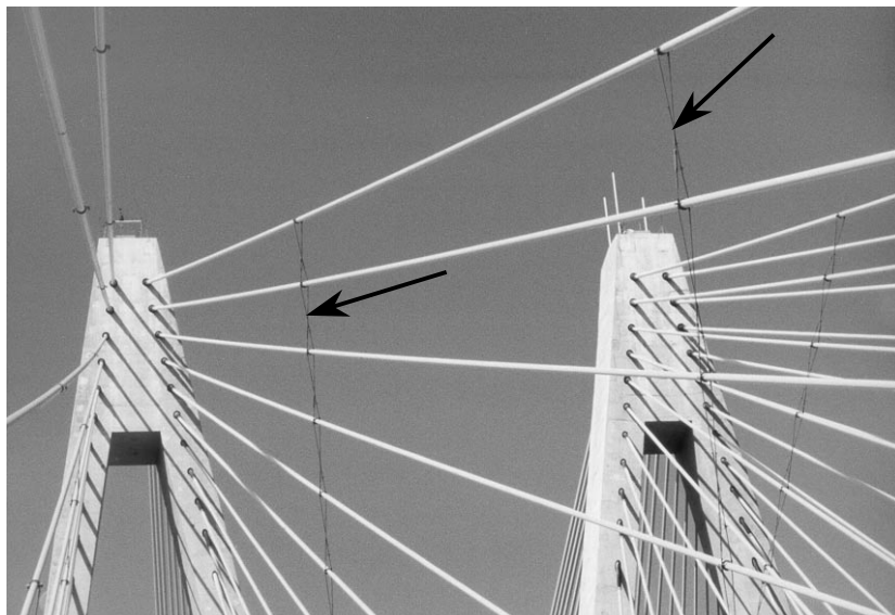
Figure 2.9: Cable Restrainers on the Fred Hartman Bridge
