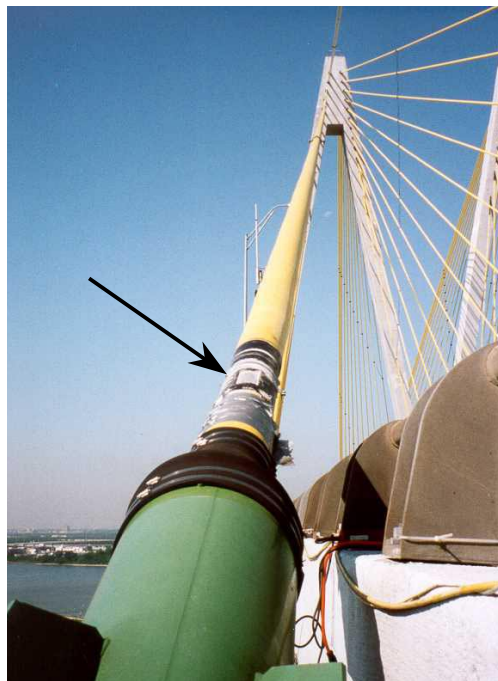
Figure 4.4: Cable A22S Showing Window in Polyethylene Sheath Where Strain Gages Were Located
