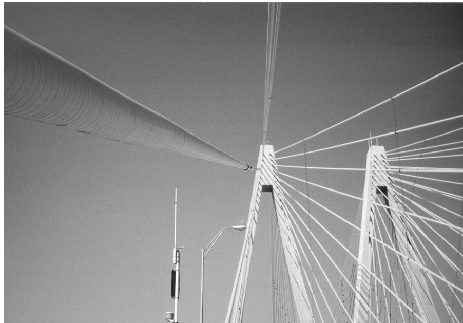
Figure 2.1: The Stay Cables of the Fred Hartman Bridge
