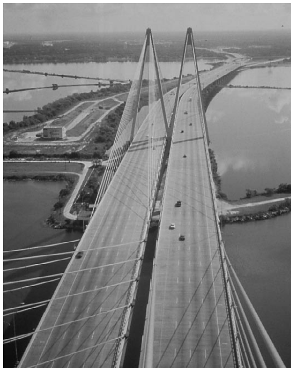
Figure 3.3: The Fred Hartman Bridge from South Pylon
