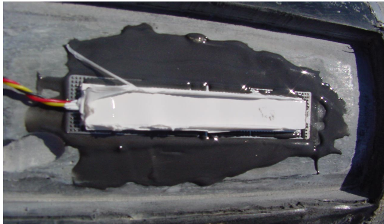
Figure 4.15: Encapsulated Strain Gage on Cable A22S
