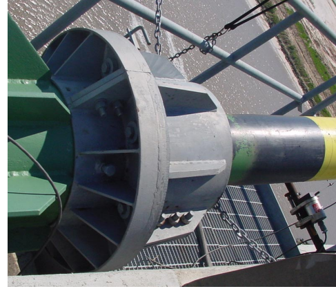
Figure 3.10: Prototype Freyssinet Damper
